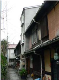
[Photo 3] A 3-story house renovated with no setback
