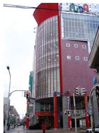
Figure 3-2 AUGA (Multiple-use facility in front of a station)
