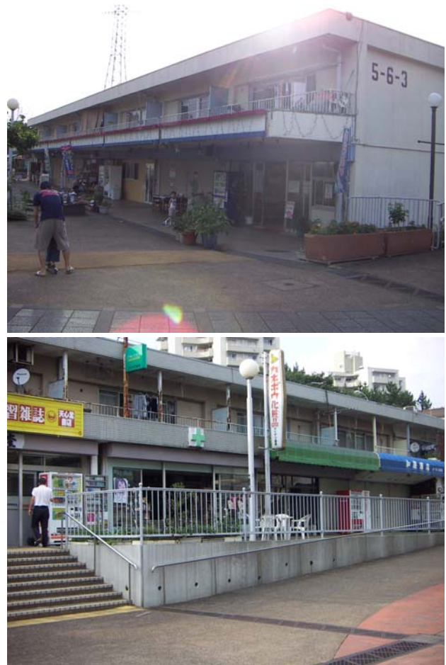
Figure-1 Suwa/Nagayama shopping mall
