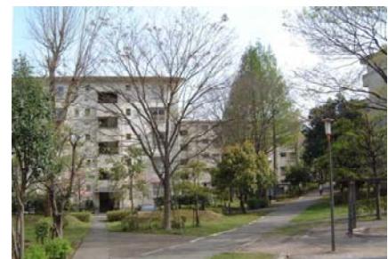
Figure-3 Apartments in good environment but small and no elevator
